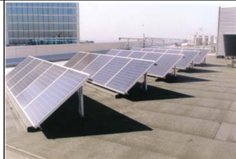
PV panels on the roof showing cast shadow
