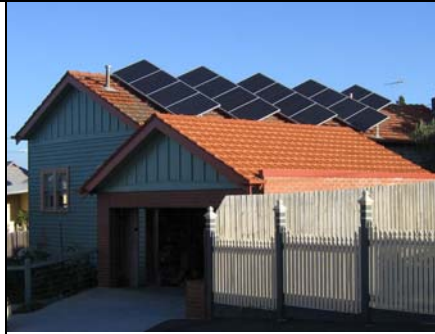
PV panels on roof
