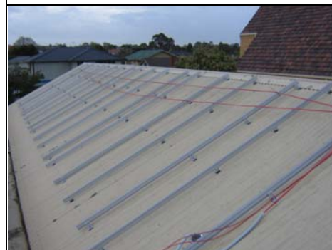
Framing Support Rails
