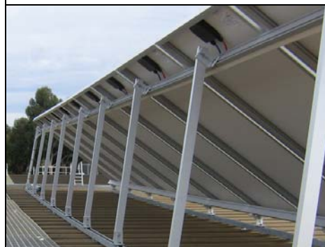
Framing Support Rails
