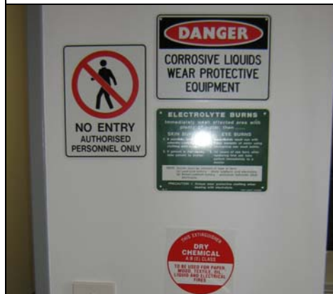
Detail of Safety Signage
