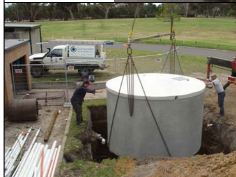
The underground water storage tank being placed into position.
