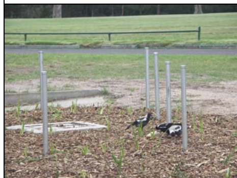
Ground above the installed water storage tank with stakes to restrict traffic.
