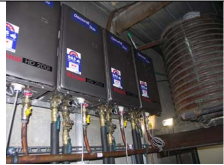
The instantaneous gas boosting bank and existing header tank.
