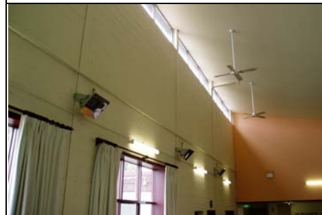
High ceilings and heating problems (Note the lights on in the daytime)
