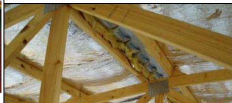
Foil and bulk roof insulation
