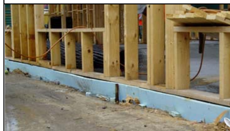
Slab-edge insulation
