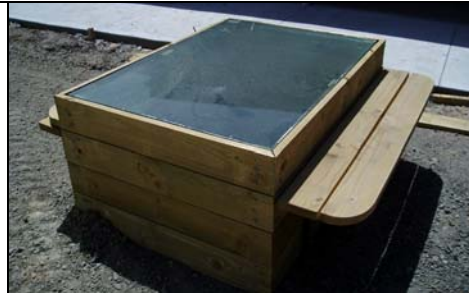
Observation window for the underground water storage
