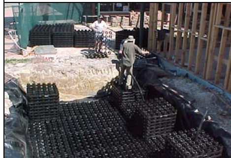
Installing the Rainstore system
