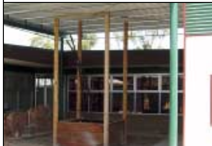
The 'cool garden' & air intake pipes
