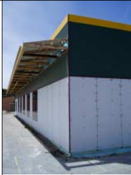
Reverse Brick Veneer and the Solar Eave – Note the shadow on 25 th Dec.
