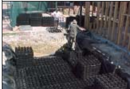
Installing the Rainstore system
