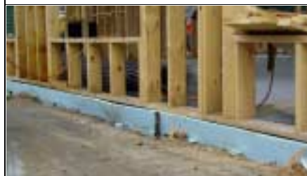
Slab-edge insulation
