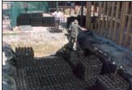
Installing the Rainstore system
