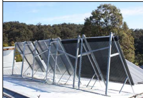
Rear of SHW Panels on Roof
