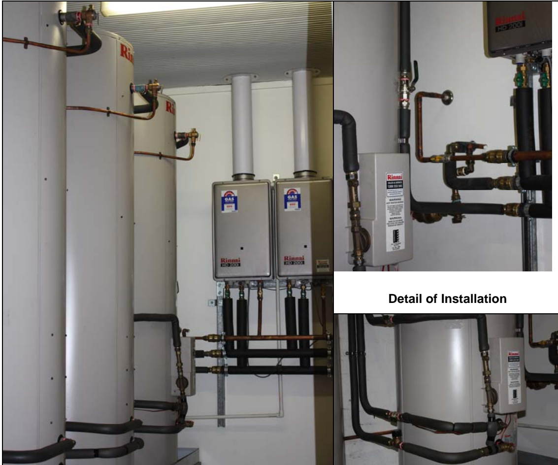
Storage Tanks and Gas Boosters
