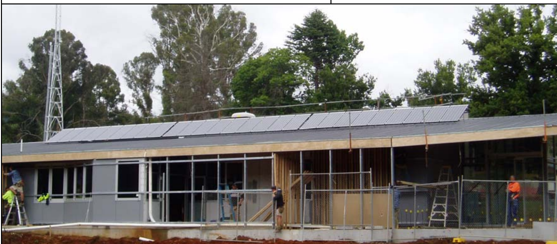
Marysville Police Station (during construction) with the PV panels installed
