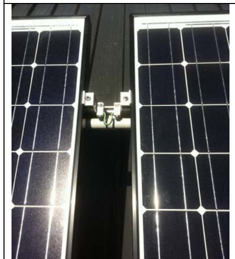
Detail of Earthing Connection
