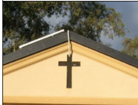
PV Cables through the Cross
