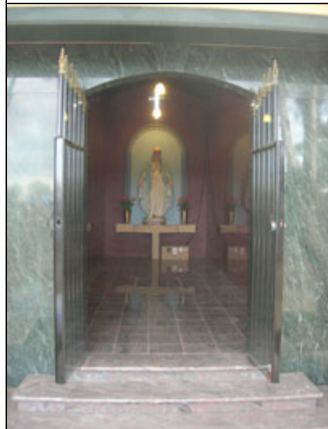
Lighting and Battery/Control Box inside the Mausoleum
