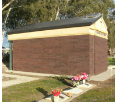
Panels on Upper West Corner of Concrete Roof
