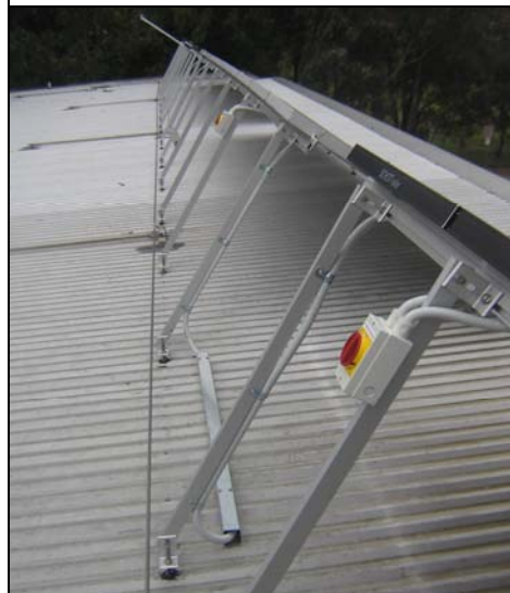
Framing Support Rails, Conduit and Isolation Switches
