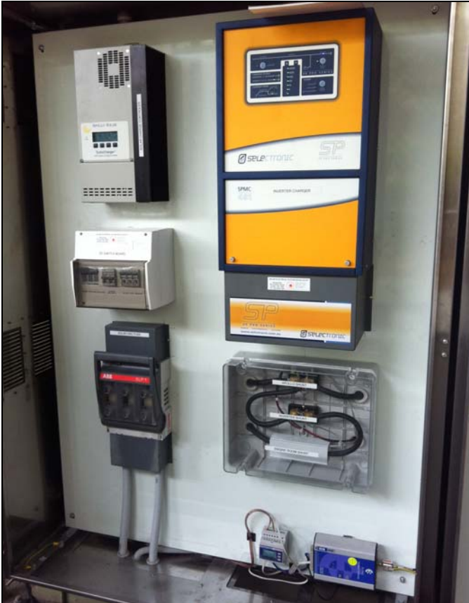
Inverter Cabinet (outer door open)
