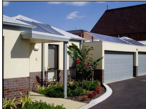
Solar Hot Water & PV Panels
