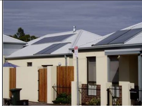
Solar Hot Water and Photovoltaic panels – note the neat appearance and absence of roof tanks
