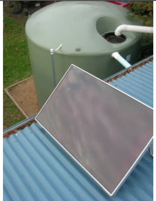
System from Shed Roof
