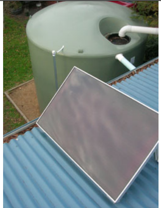
System from Shed Roof
