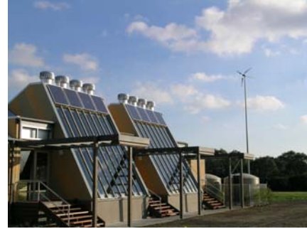
View of Solar Chimneys and Wind Turbine
