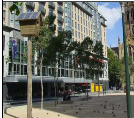
PV panels on the roof
