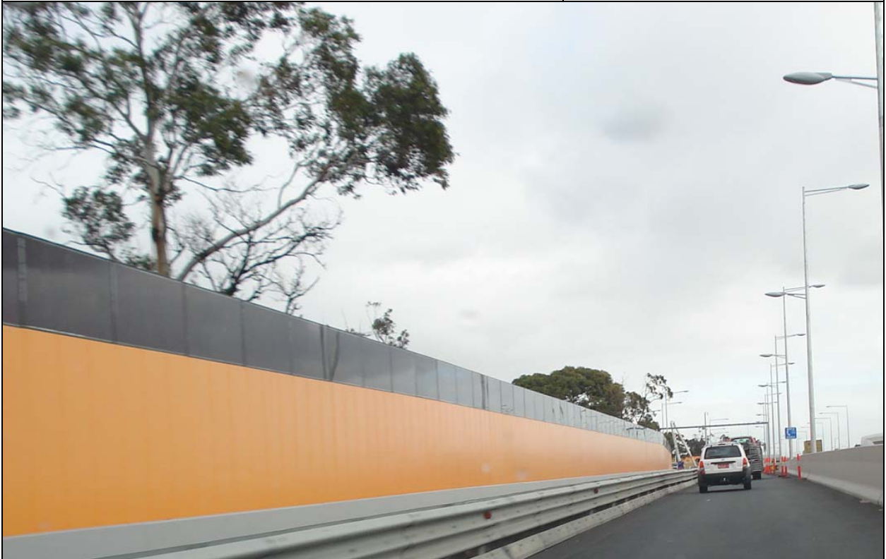
The Freeway Side of the Wall
