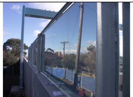
Bicycle Path at Rear of Array
