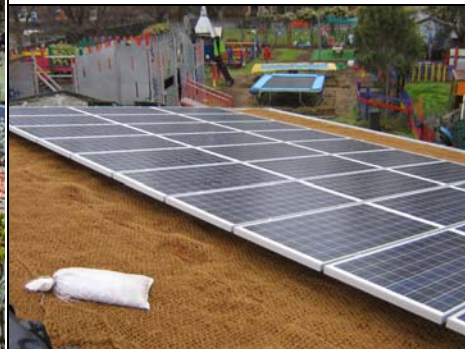
Solar Panels Installed
