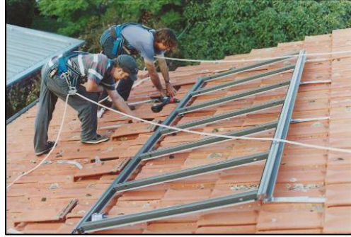
GS Contractors with safety harnesses
