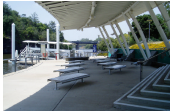
RiverCat Wharf at Parramatta
