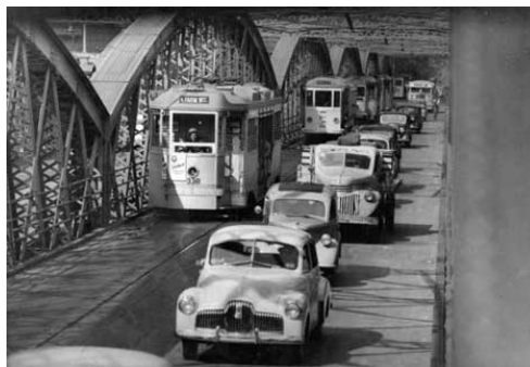
Cars and trams travelling along Victoria Bridge, Brisbane, 1952 Photo: State Library of Queensland
