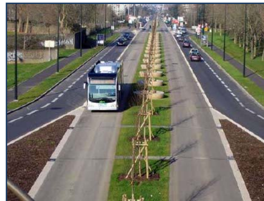
BusWay. Nantes, France Photo: D Peña
