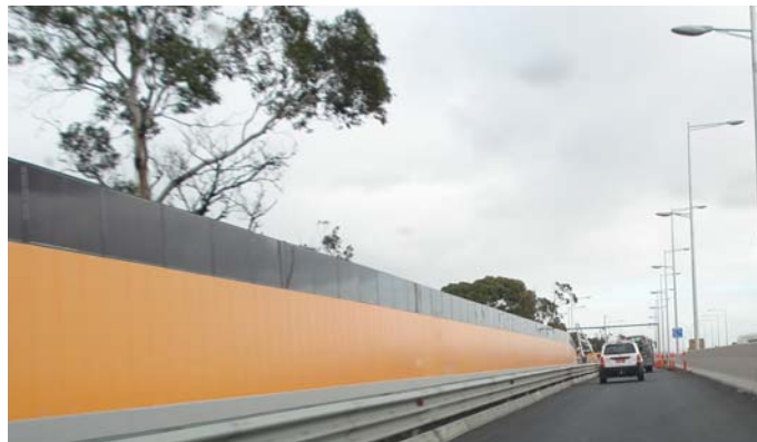
Solar Noise Wall (installed by Going Solar) on the Tulla-Calder Interchange Picture: Warwick Johnston
