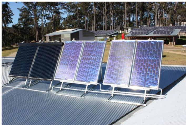
Evacuated tubes on the left hand side and flat plate panels on the right. (PV panels are on the roof in the background)
