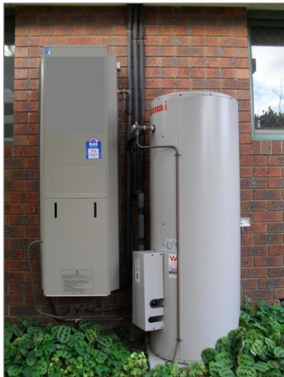
Existing gas-boostered storage tank on the left coupled with a new solar storage tank on the right. (The more storage the better).
