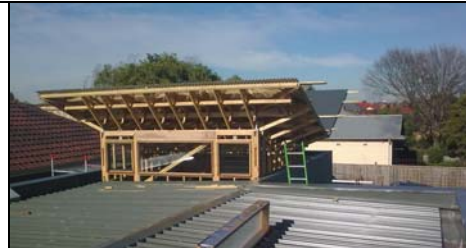
Butterfly Roof (under construction)
