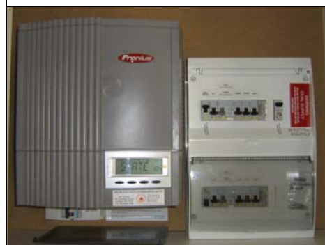
Inverter & Switchboard
