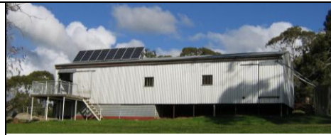
PV Panels on the Shed Roof
