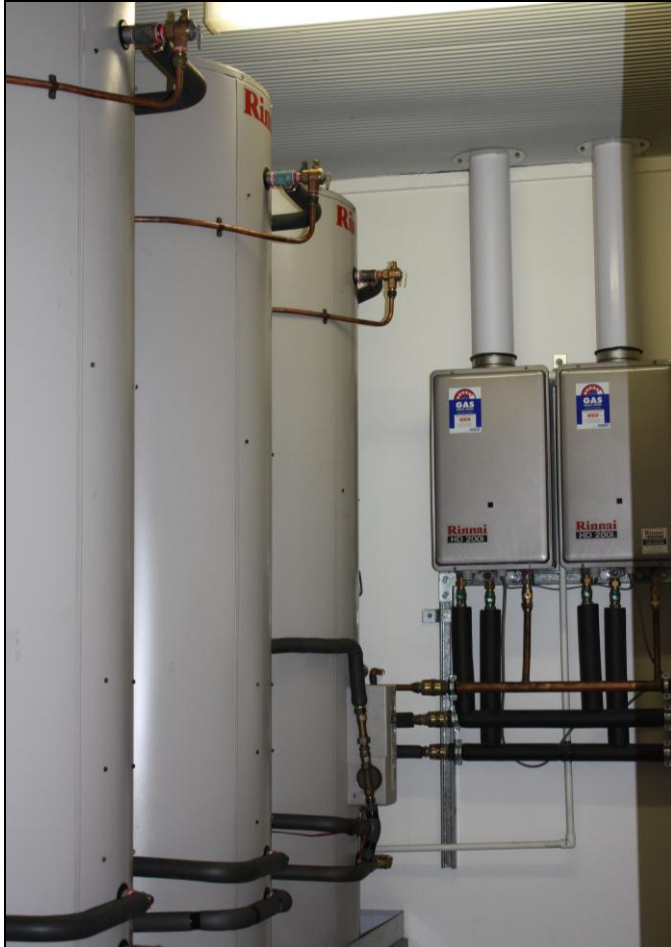
Storage Tanks and Gas Boosters
