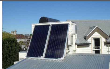
SHW Panels on Roof
