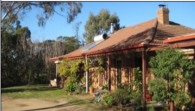
The house with the solar hot water system
