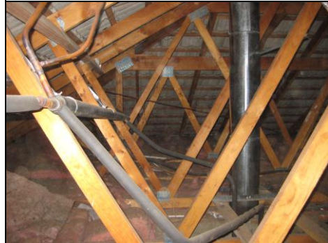
Inside the roof showing the Tedson heat exchanger (centre left and the wood stove flue (centre right)
