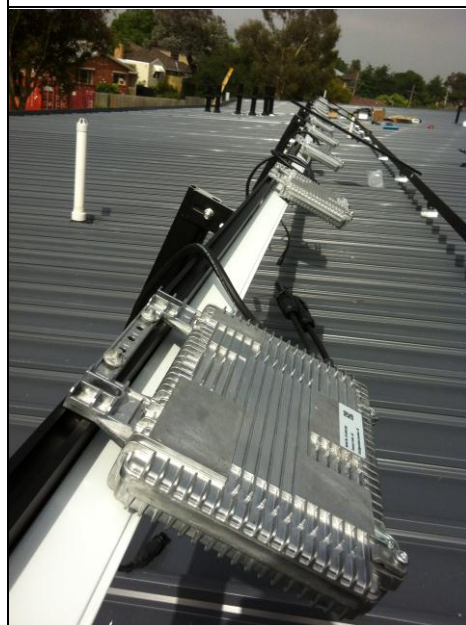
Micro-Inverters on framing before the PV panels are installed.
